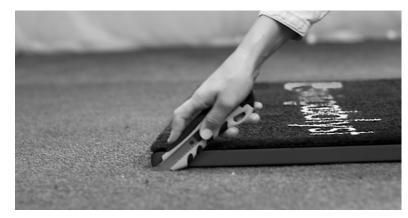
1 Cut a hole in the turf matching the Balance Plate dimensions (see page 13) so it becomes a tight fit.
